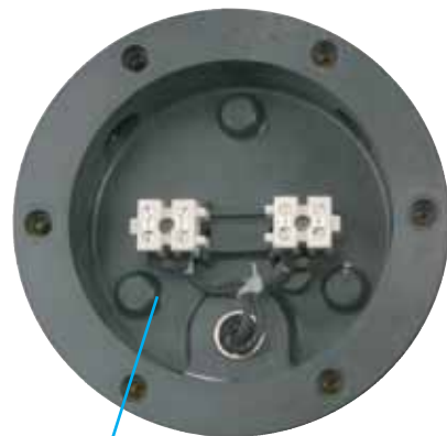
terminal connection chamber „e“
